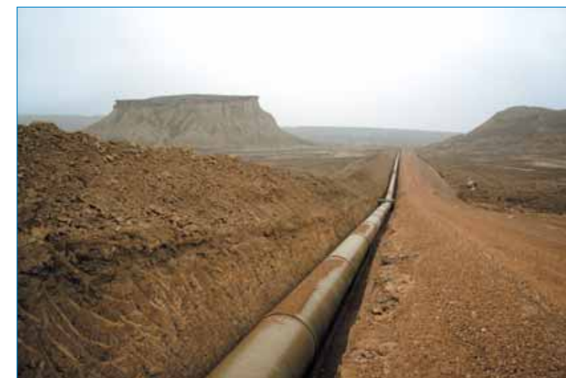
Completed part of Oguz-Gabala-Baku water pipeline
